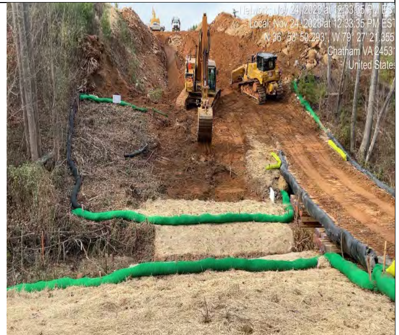
Photo Description: Restoration of the 50-foot buffer on the CIS.
