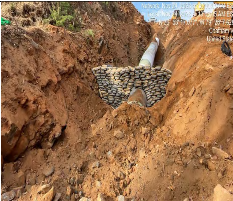
Photo Description: The CIS trench breaker after installation.
