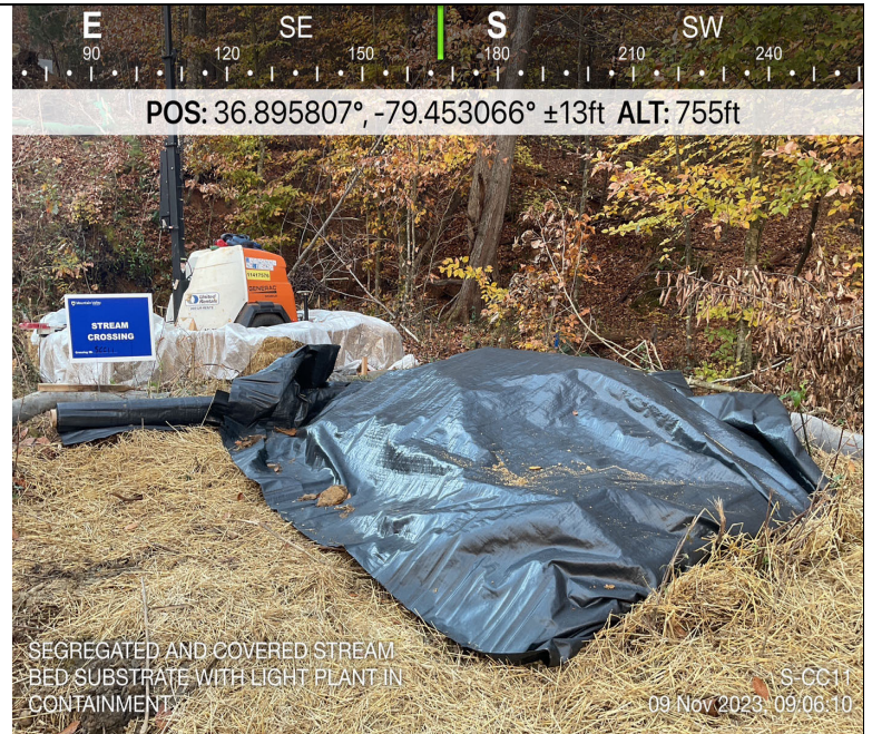
Photo Description: Segregated and covered stream bed substrate.
