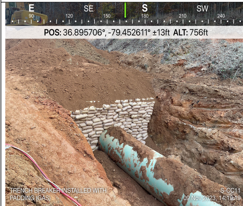
Photo Description: Trench breaker installed (GAS).
