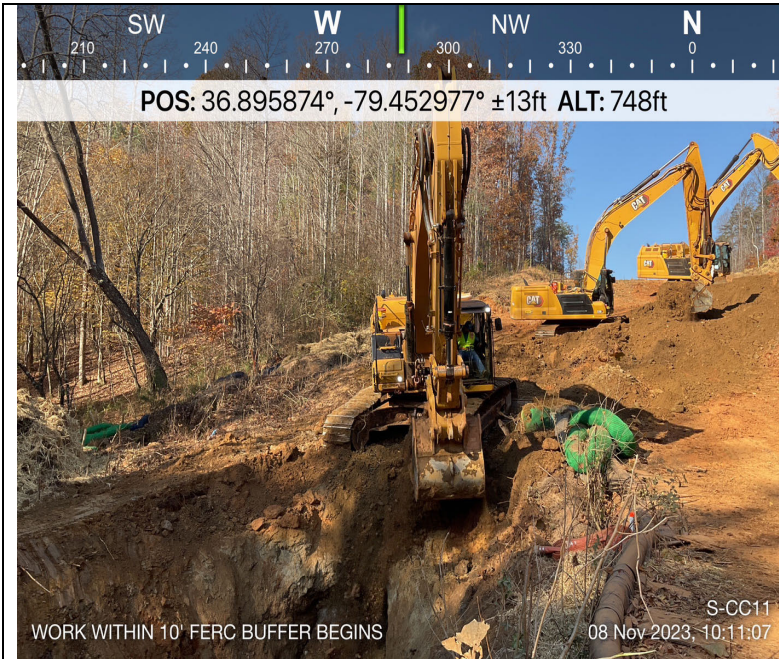
Photo Description: Crossing construction begins within 10' FERC buffer.
