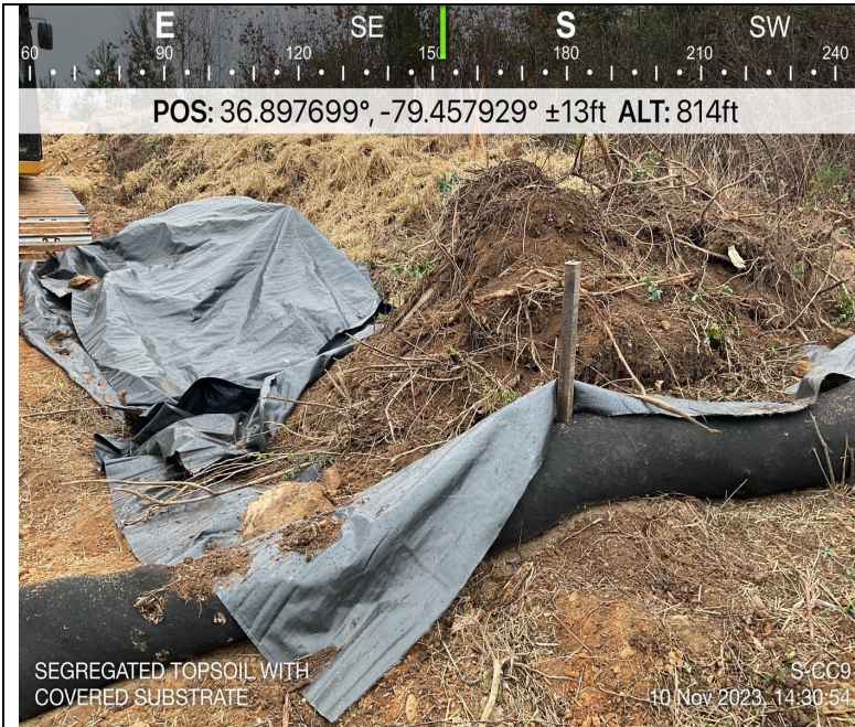
Photo Description: Segregated topsoil and stream bed substrate enclosed in geotextile fabric.
