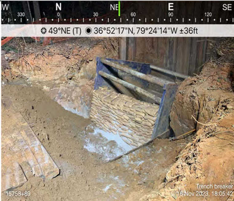
Photo Description: A trench breaker after installation and during subsoil backfill.
