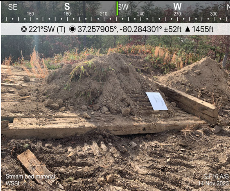
Photo Description: Top 12" of streambed substrate segregated and stockpiled separately.
