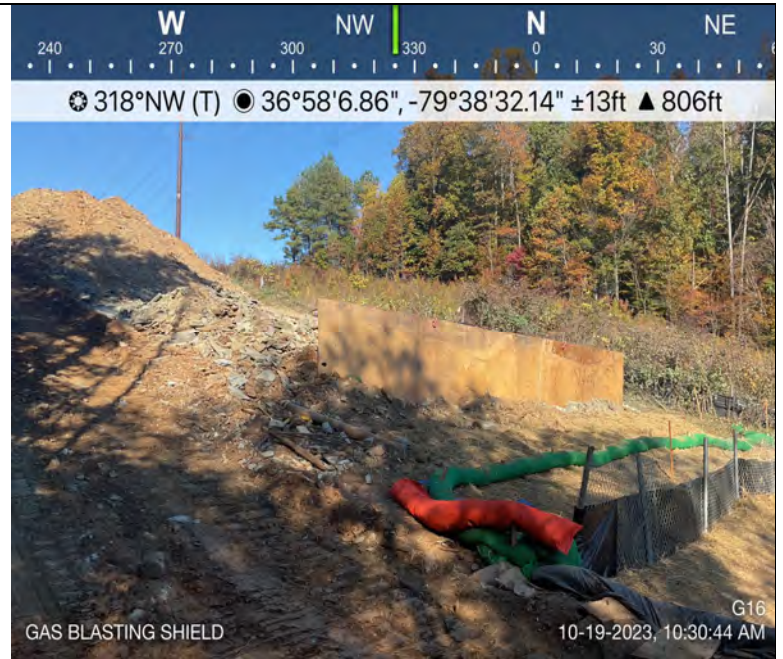
Photo Description: Stream protection installed for blasting activities.
