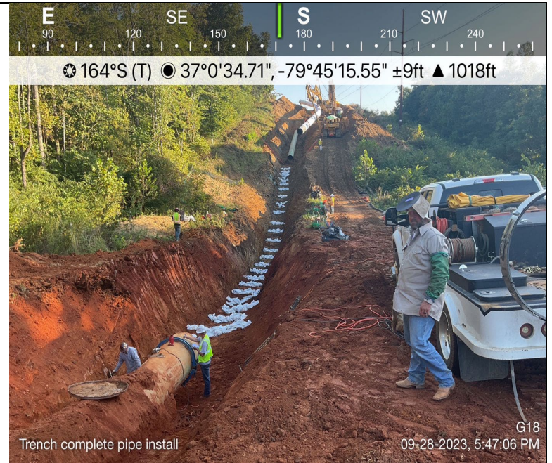
Photo Description: Trenching overview
