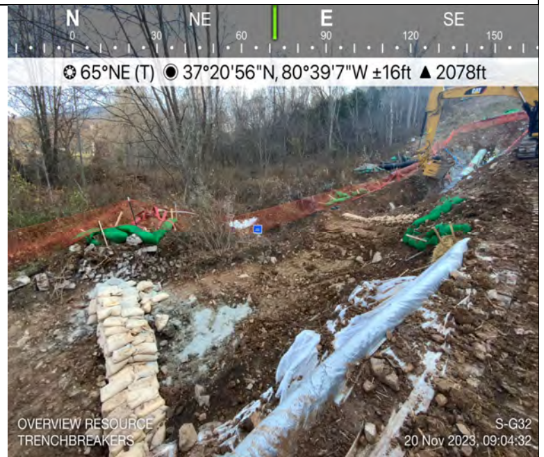
Photo Description: An overview of the trench breakers after installation.
