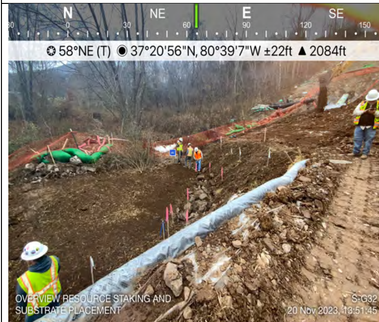
Photo Description: The survey crew providing guidance for stream substrate replacement.
