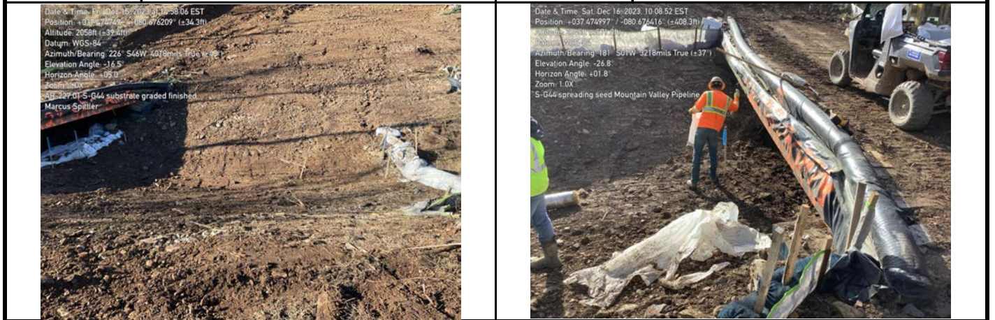
GPS Location See Photo GPS Location See Photo Description Photo 7: Substrate added and channel contoured. Description Photo 8: Seeding buffer.
