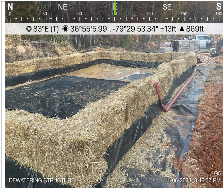
Photo Description: Dewatering structure for bags and sediment control.
