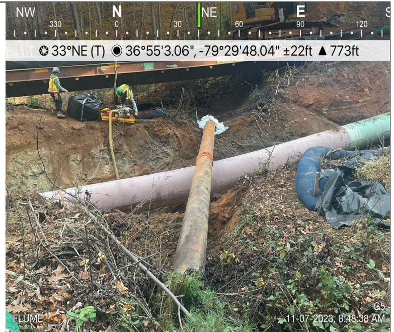
Photo Description: Flume installed throughout crossing.
