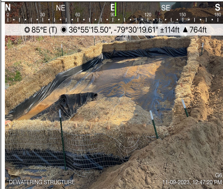
Photo Description: Dewatering Structure
