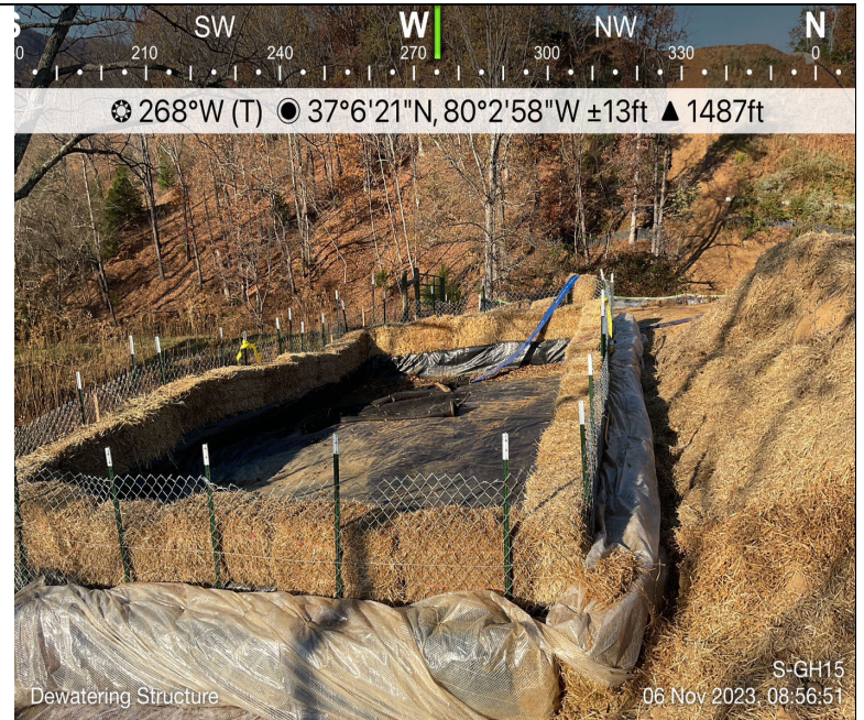
Photo Description: Dewatering structure on-site throughout crossing.
