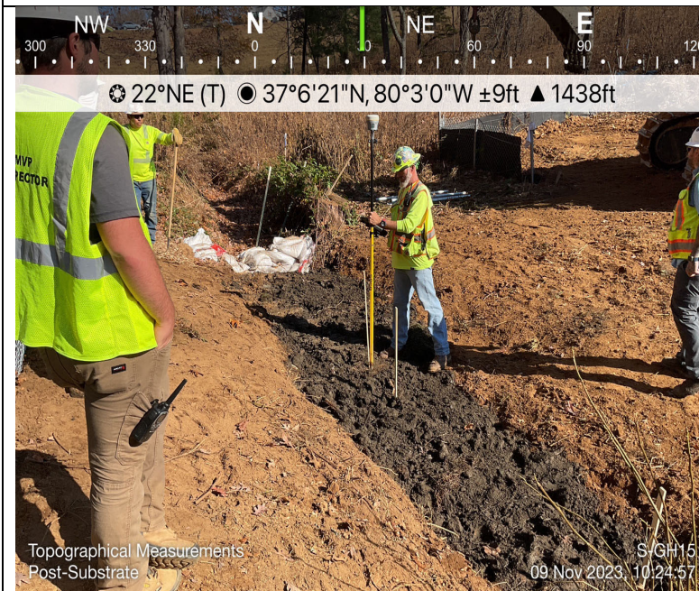
Photo Description: Survey on-site assisting with restoration.
