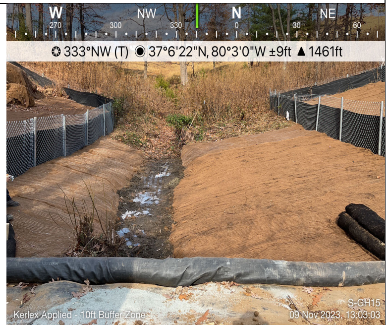
Photo Description: Erosion control matting Installed in buffer zones.
