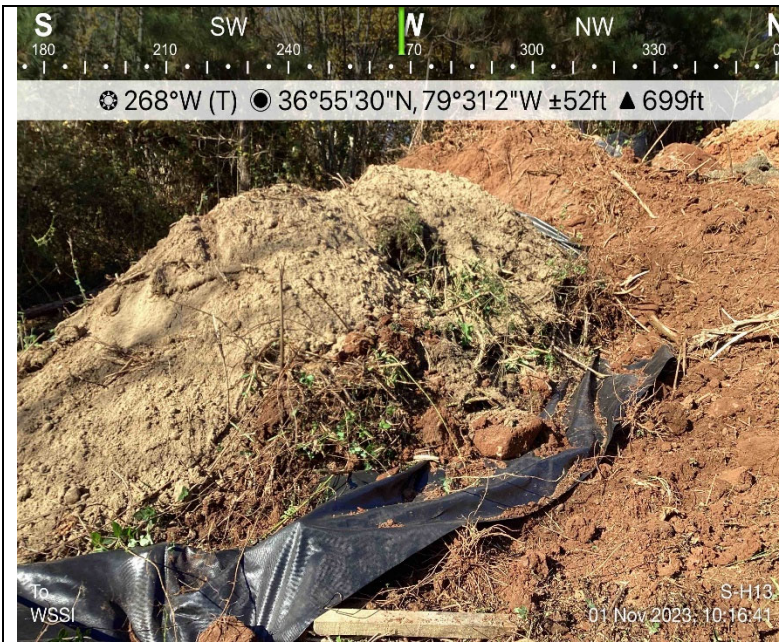
Photo Description: Topsoil stockpiled separately and stabilized.
