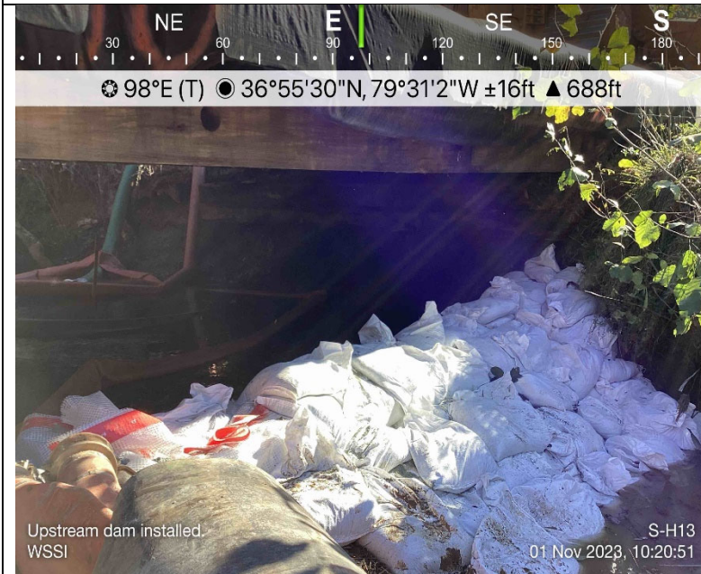
Photo Description: Upstream dam installed and functional throughout crossing.
