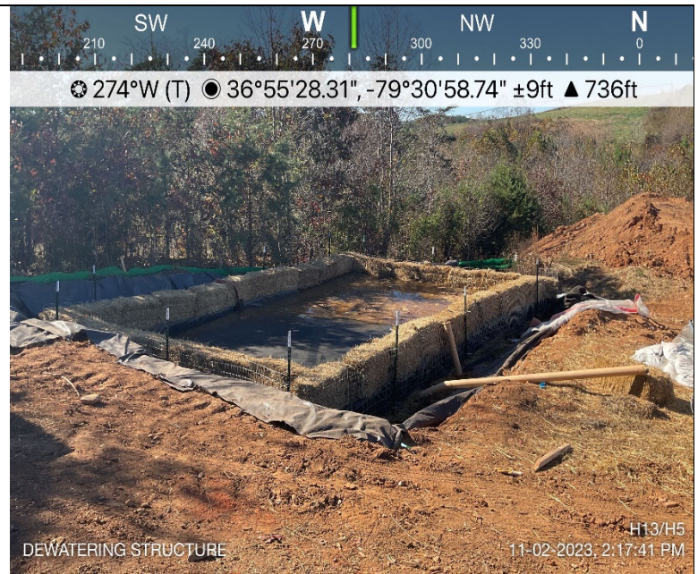
Photo Description: Dewatering structure installed for throughout crossing.
