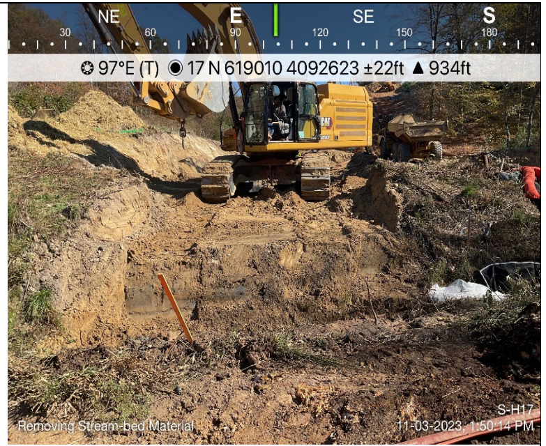
Photo Description: Excavation of the streambed.
