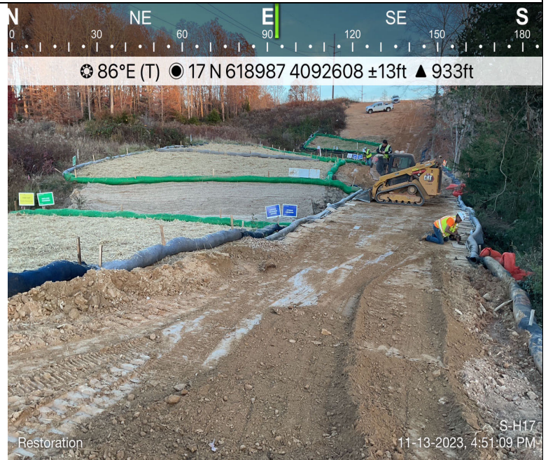
Photo Description: Site restoration and installation of the filter sock.
