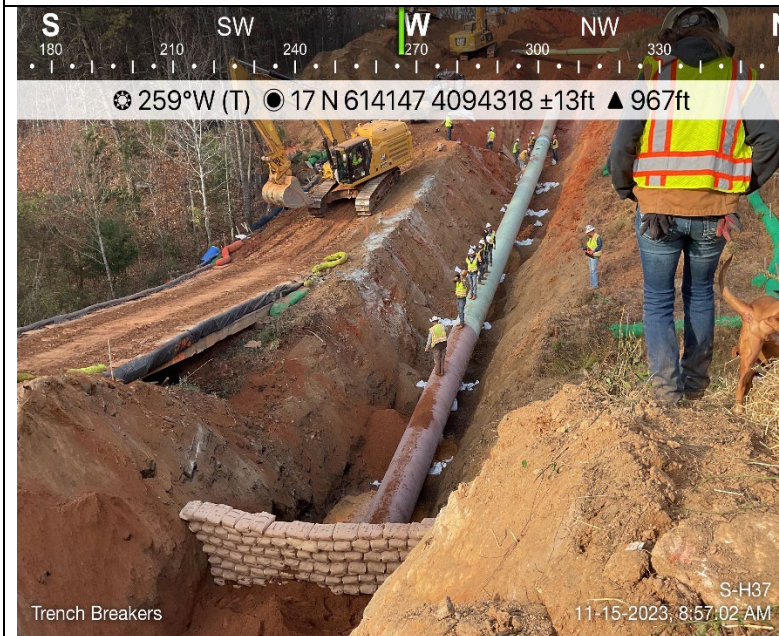
Photo Description: A trench breaker after installation.
