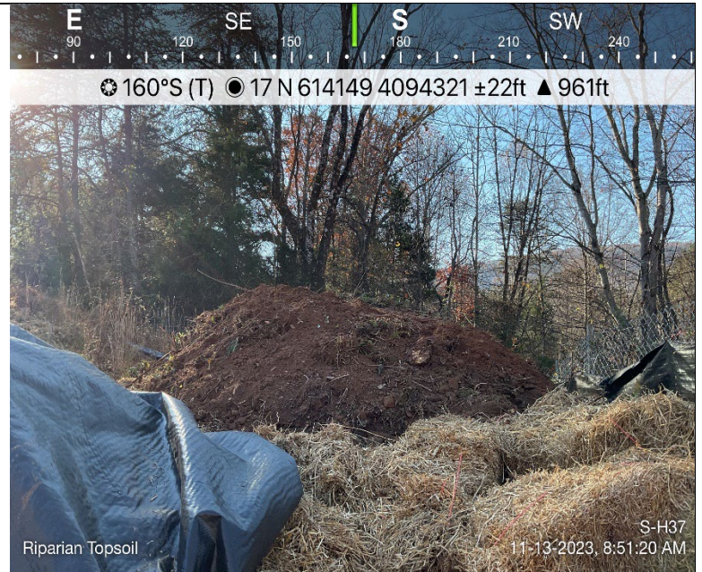
Photo Description: The topsoil has been segregated and stockpiled.
