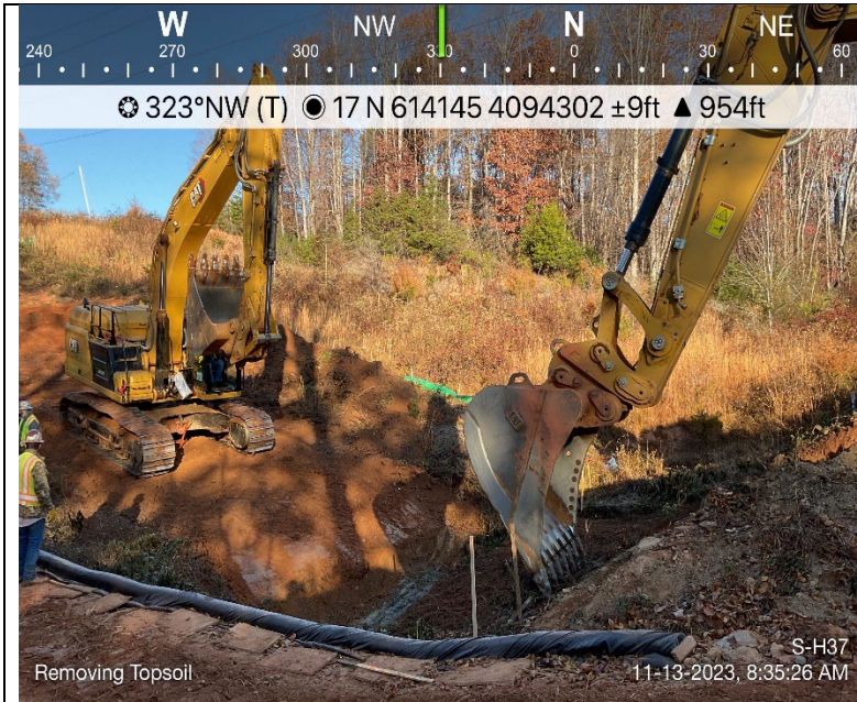
Photo Description: Excavation of the topsoil.
