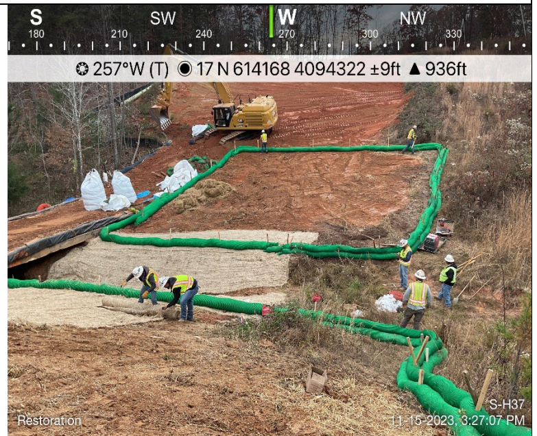
Photo Description: The environmental crew installing straw matting during restoration.
