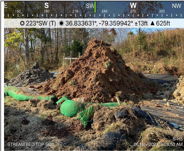
Photo Description: Stream bed topsoil stockpiled separately on geotextile fabric.
