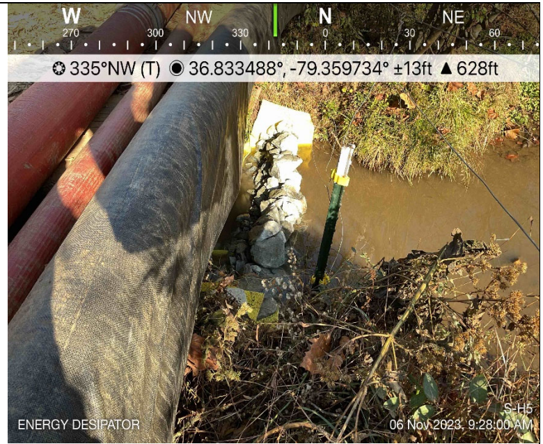
Photo Description: Energy dissipator installed and operating for pump around.
