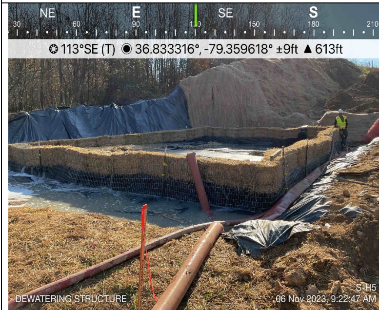
Photo Description: Dewatering structure installed and operational throughout crossing.
