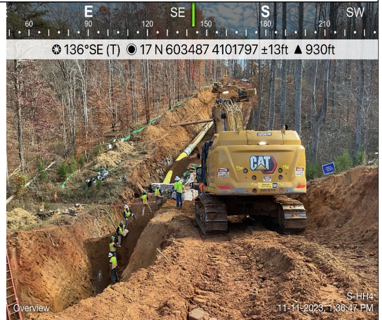
Photo Description: The crew installing a trench breaker.
