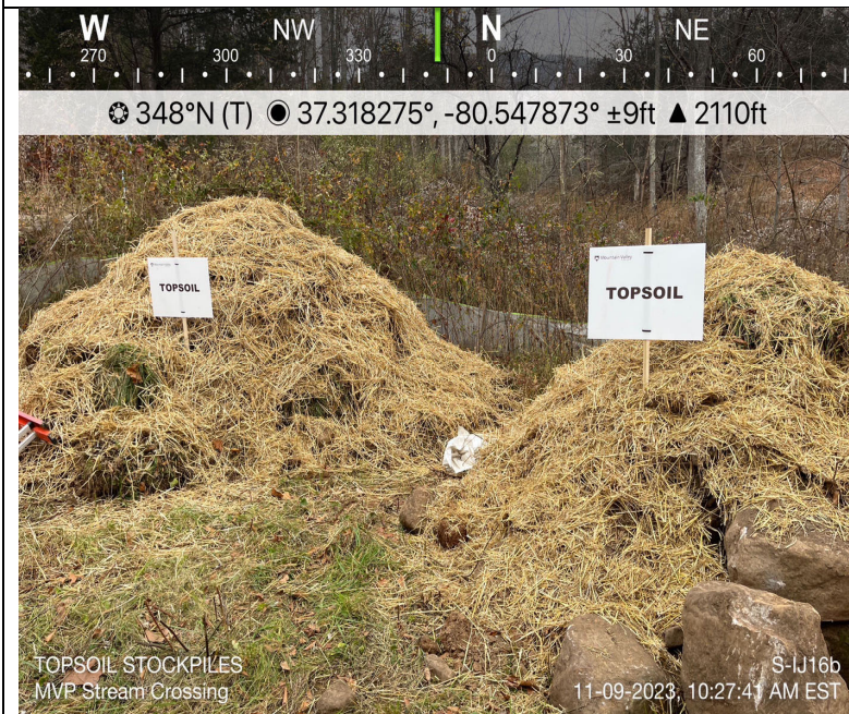
Photo Description: Topsoil stockpiles
