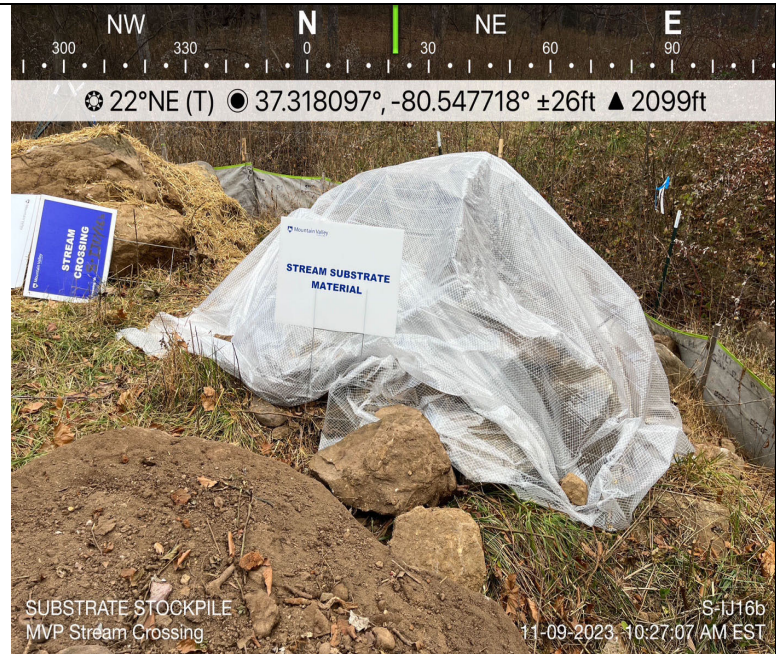
Photo Description: Stream substrate stockpile
