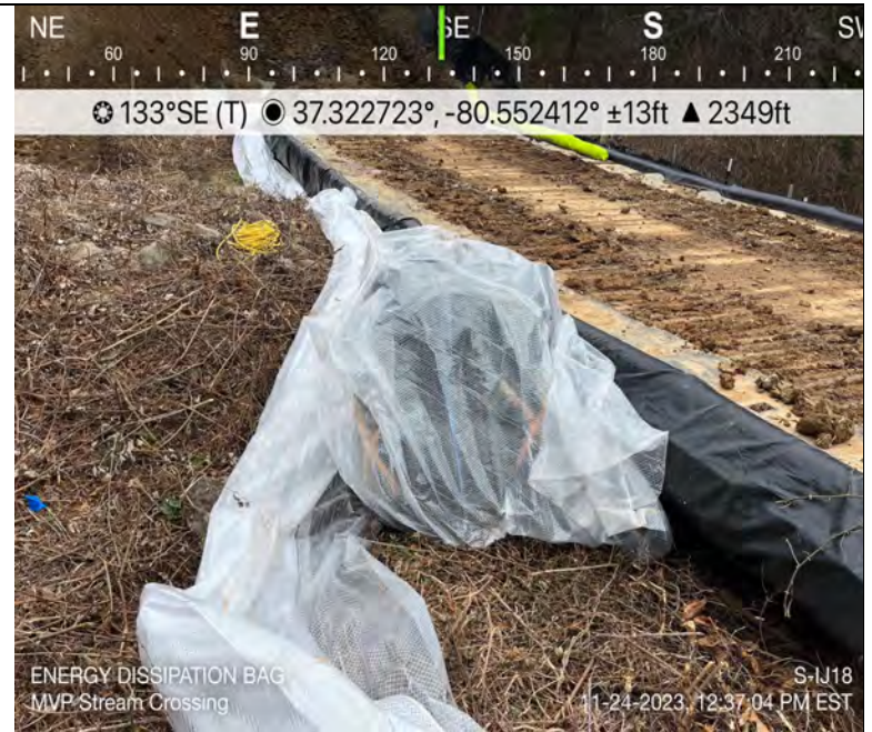
Photo Description: Energy dissipator (covered in plastic).
