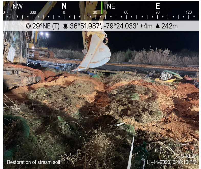
Photo Description: The stream bed soil was replaced. The resource was restored.
