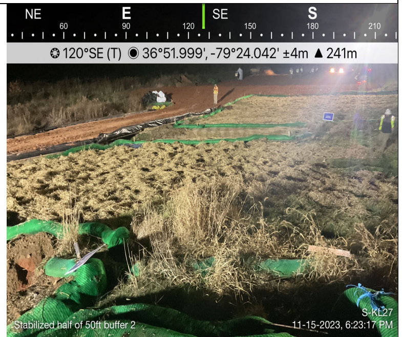
Photo Description: The 50 foot buffer was seeded and stabilized with straw.
