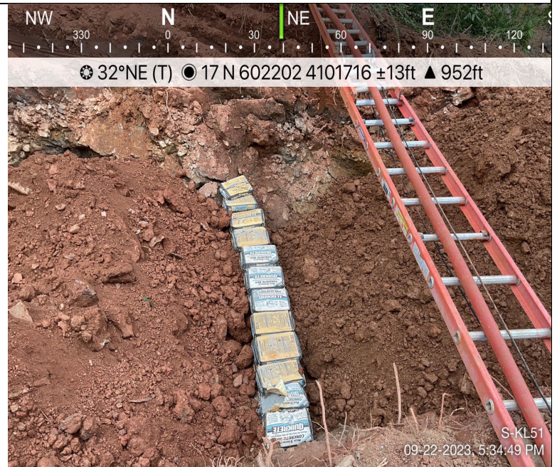
Photo Description: A trench breaker after installation.
