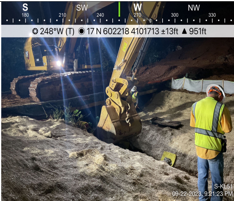
Photo Description: Stream substrate and cobble being returned to the stream bed.
