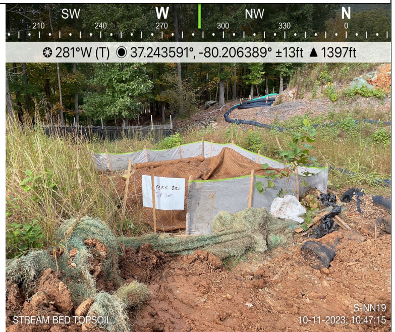
Photo Description: Stream substrate/topsoil stockpiled and stored separately from subsoil.
