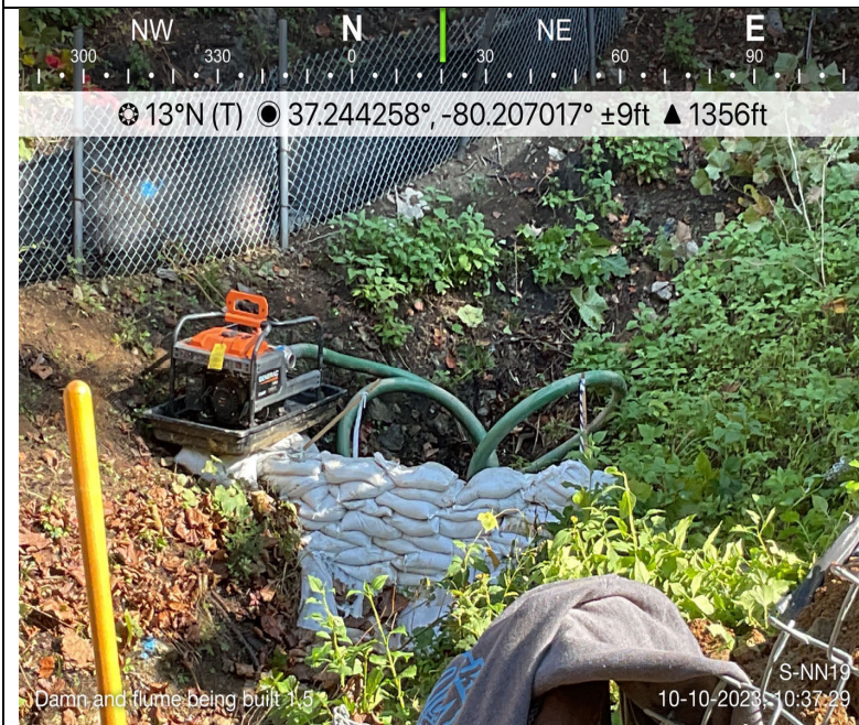
Photo Description: Dam and pump installed and operation during crossing activities.
