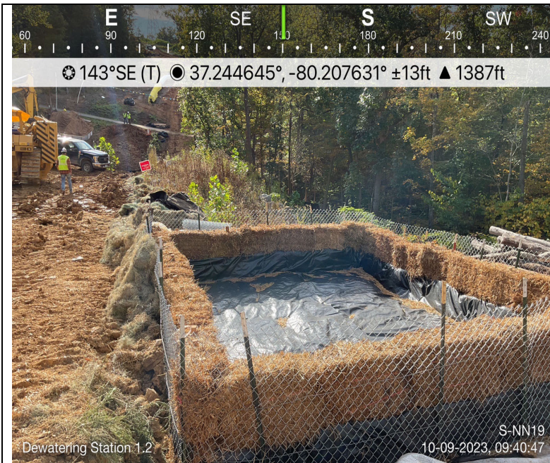
Photo Description: Dewatering structure installed and operation during crossing.
