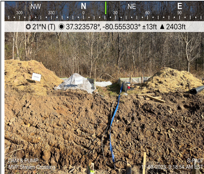
Photo Description: Dam & pump
