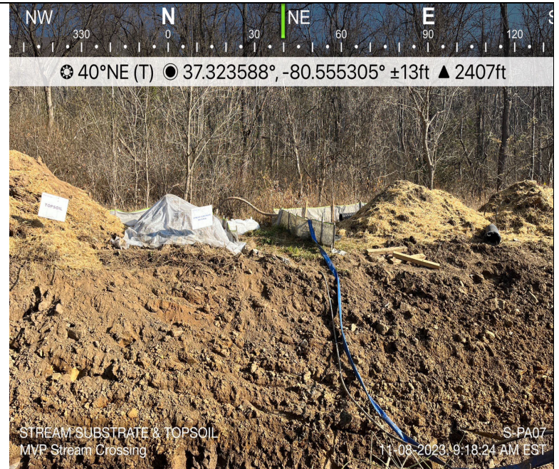
Photo Description: Soil stockpiles
