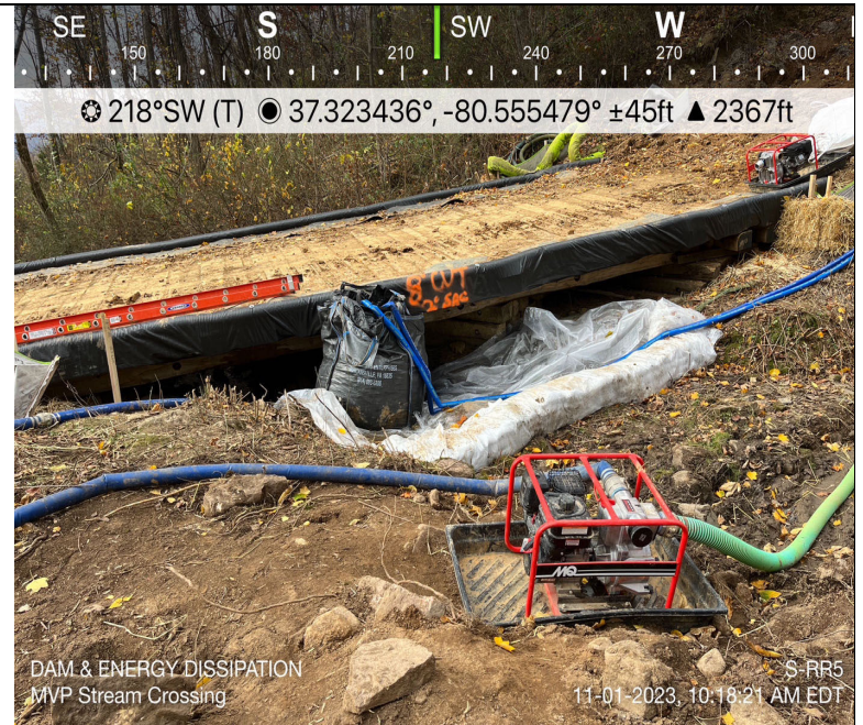
Photo Description: Dam & energy dissipation bag
