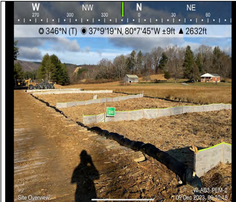
Photo Description: Site overview after restoration activities.
