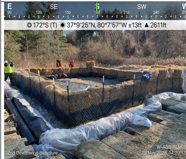
Photo Description: Second dewatering structure installed to assist with trench dewatering.
