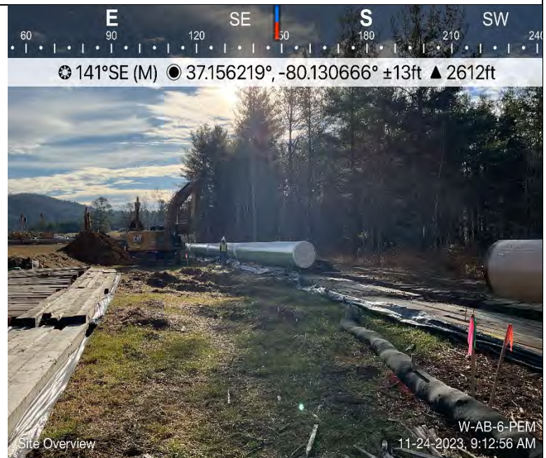
Photo Description: Site overview of upland activities outside resource impact area.
