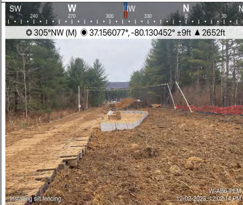
Photo Description: Erosion and sediment controls installed around re-stored wetland area.
