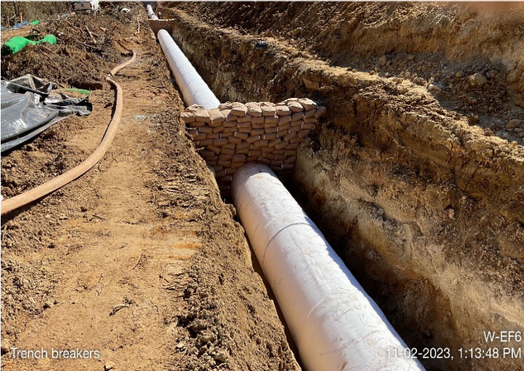
Back filling with padded soil
