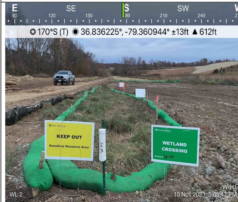
Photo Description: Wetland W-H1 avoided by construction.
