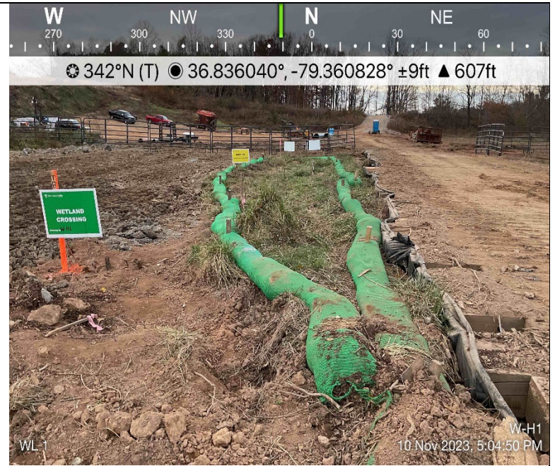
Photo Description: Wetland area avoided by construction.
