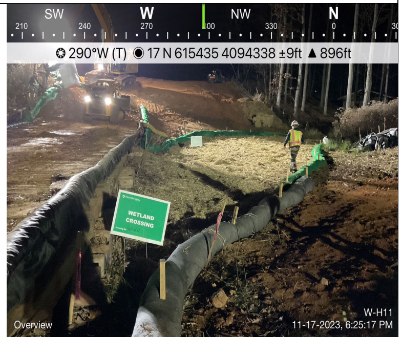
Photo Description: Overview of the resource during restoration activities.
