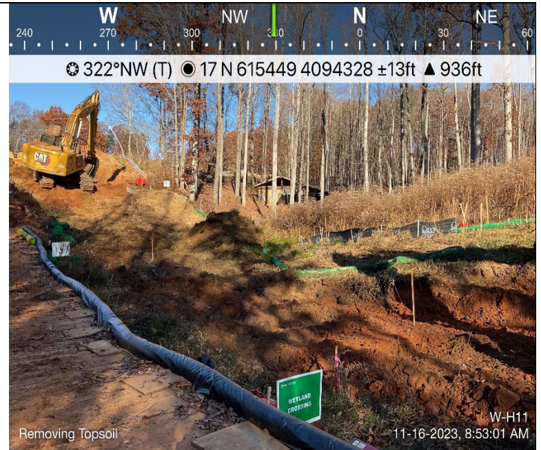
Photo Description: Topsoil being removed from the resource.
