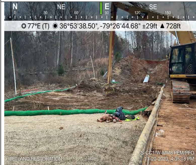
Photo Description: Restoration of soil to the wetland impact area.
