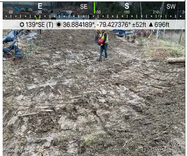
Photo Description: Seed being applied after restoration of the topsoil.
