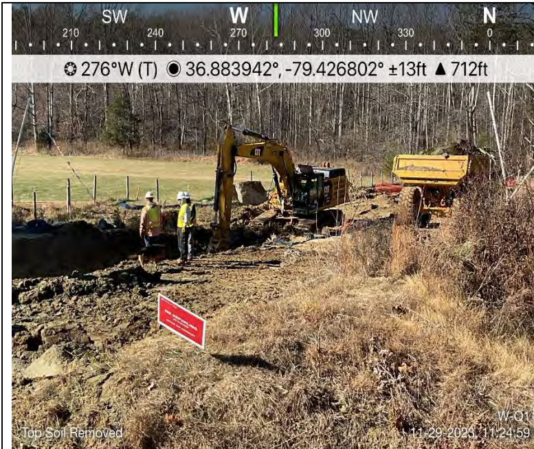
Photo Description: Topsoil being excavated from the trench.
