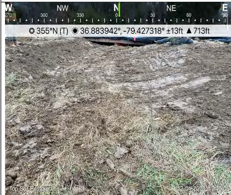
Photo Description: Topsoil restored within the resource.
