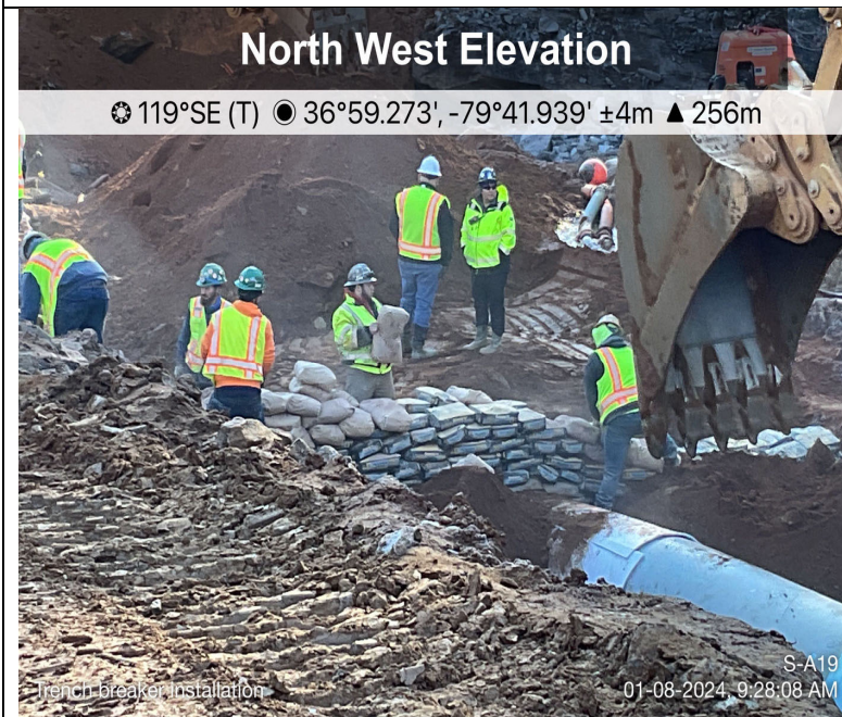
Photo Description: Trench breaker installation.
