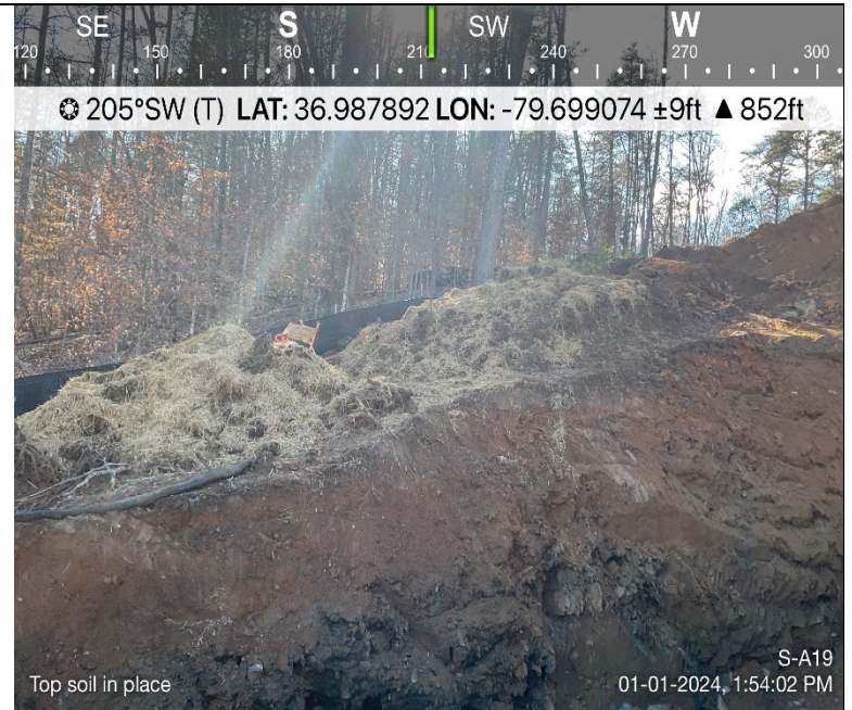
Photo Description: The topsoil was stockpiled and stabilized with straw mulch.
