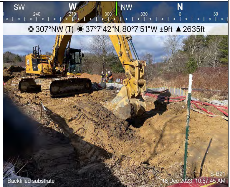
Photo Description: Backfilling of the stream substrate.
