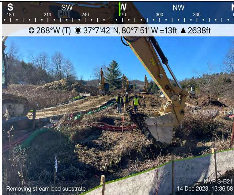
Photo Description: Excavation of the streambed substrate.
