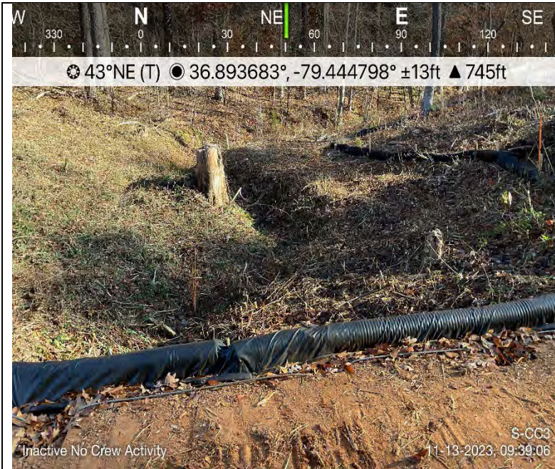
Photo Description: Upstream view of permitted impact area during pre-construction assessment.
