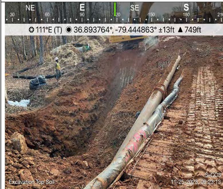
Photo Description: Topsoiling and Trench Excavation
