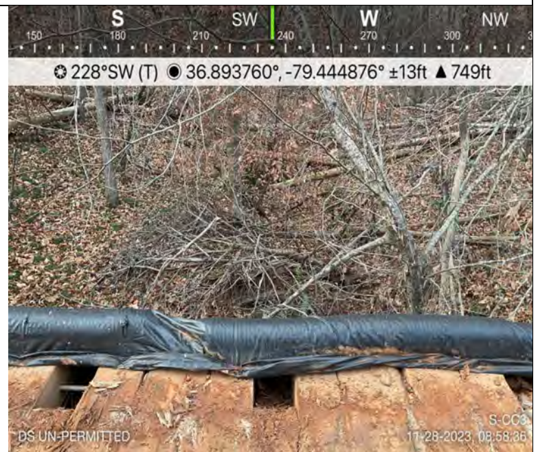
Photo Description: Conditions of the downstream area outside the ROW during post-construction assessment.
