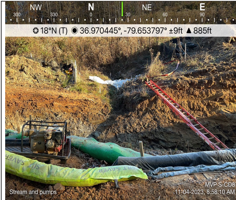
Photo Description: An overview of the dam and pump installed onsite.
