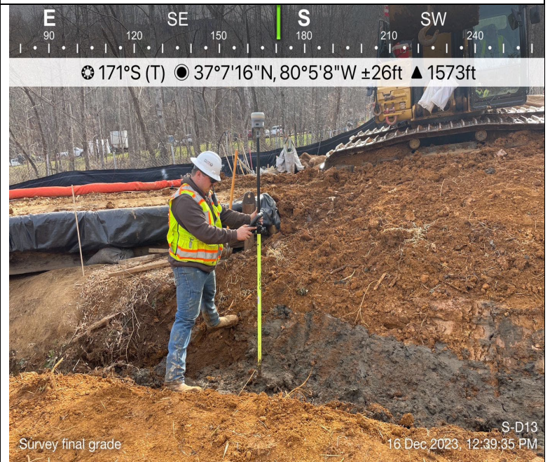
Photo Description: Survey shooting final grade for the stream bed elevation.
