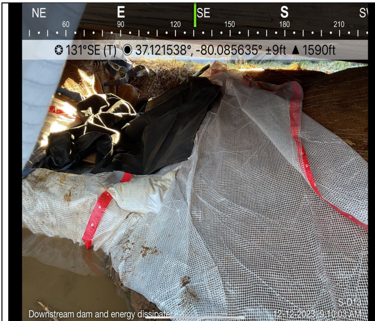
Photo Description: An overview of the downstream dam and energy dissipater.
