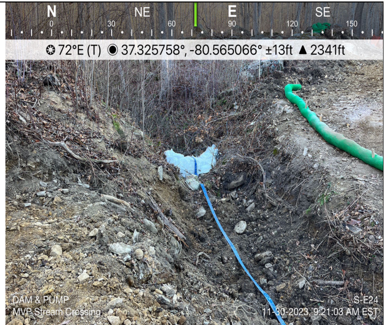
Photo Description: Dam & pump operation maintained throughout construction.
