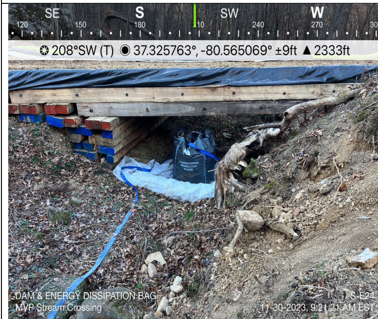
Photo Description: Downstream dam & energy dissipation bag
