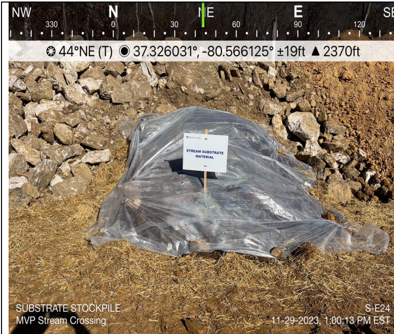
Photo Description: Stream substrate stockpile and stabilization
