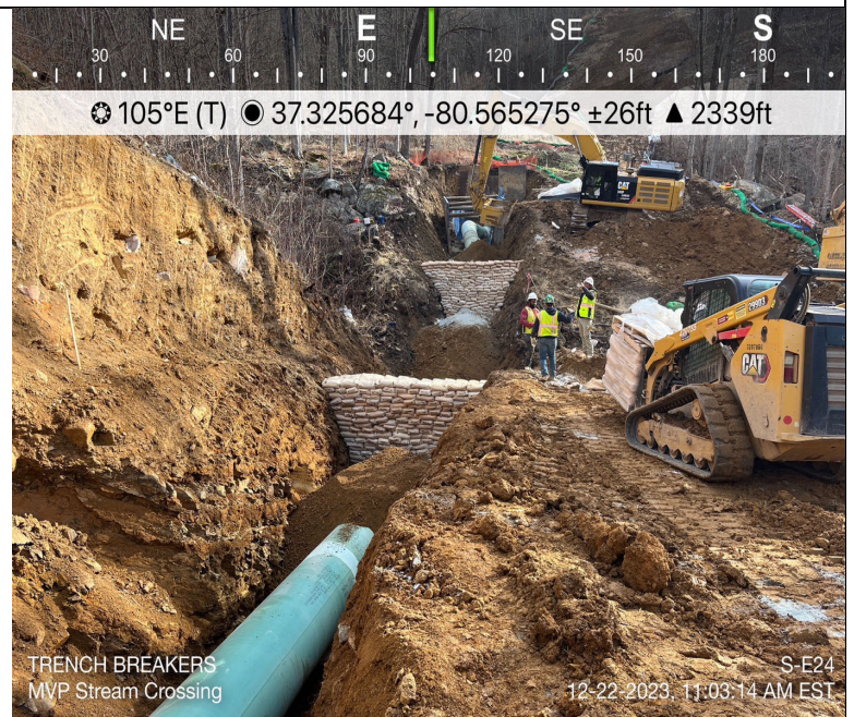
Photo Description: Trench breaker installation and subsoil padding backfill.
