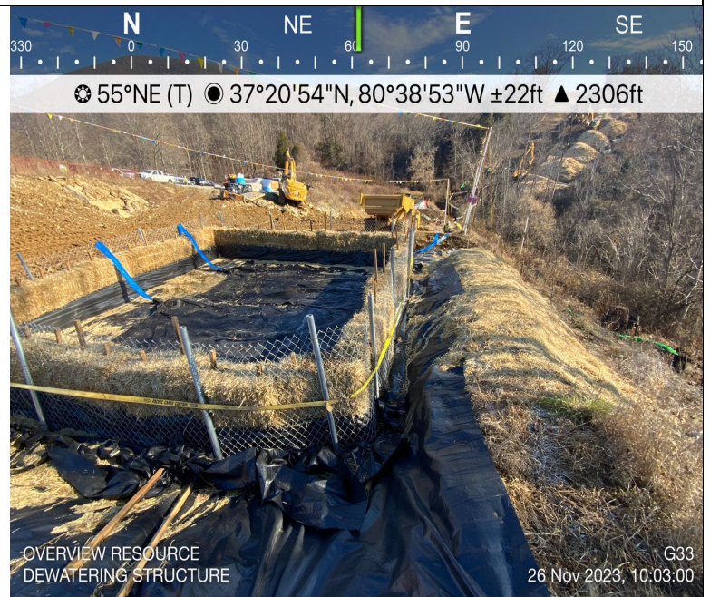
Photo Description: Dewatering structure located within the LOD.
