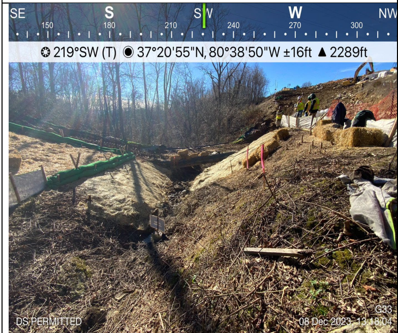
Photo Description: Downstream view of permitted impact area during post-construction assessment.
