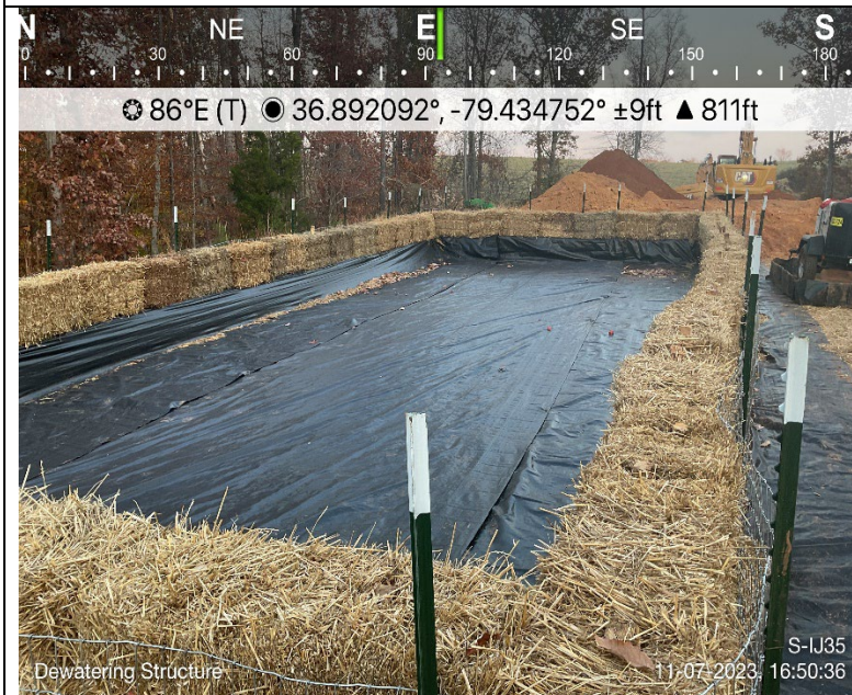
Photo Description: An overview of the dewatering structure.
