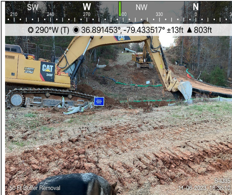
Photo Description: Excavation of the 50-foot buffer.
