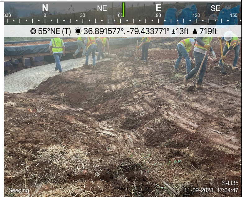
Photo Description: The crew seeding and installing straw matting.
