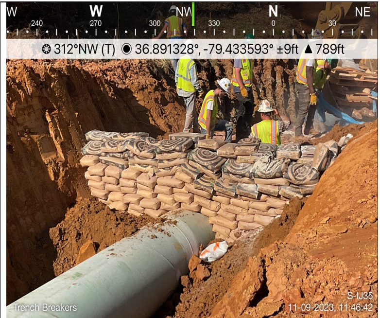
Photo Description: The crew installing trench breakers.
