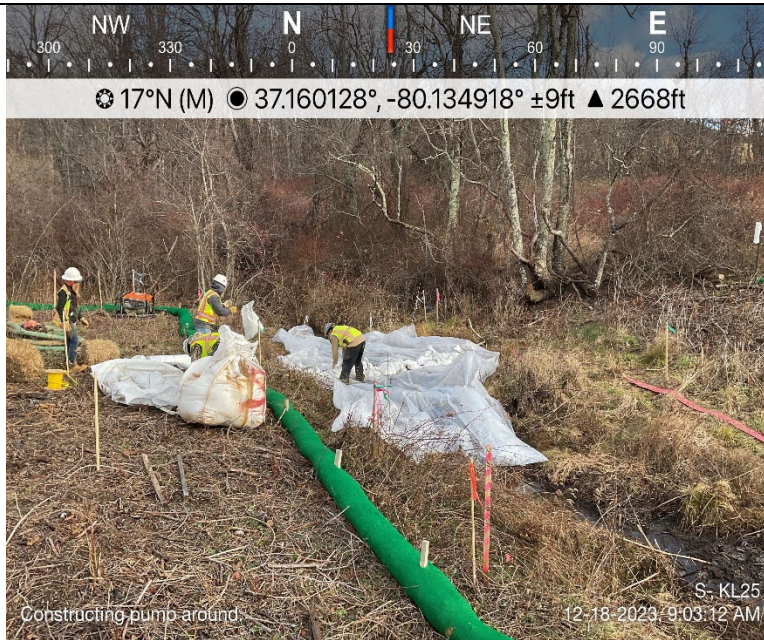
Photo Description: The construction of the pump around for the stream.
