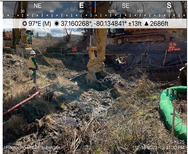
Photo Description: Excavation of the stream substrate.
