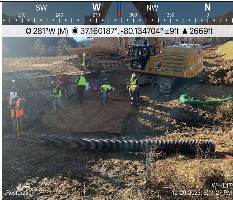
Photo Description: Restoration of the stream bank with matting.
