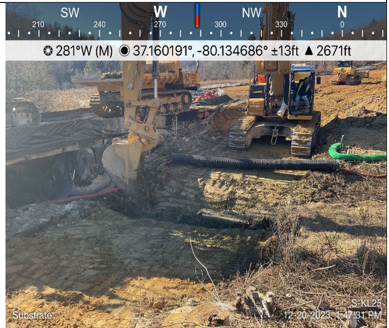
Photo Description: Restoration of the stream substrate.
