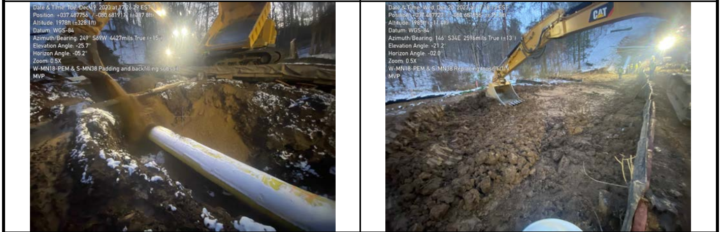
GPS Location See Photo GPS Location See Photo Description Photo 5: Backfilling. Description Photo 6: Topsoil restoration.
