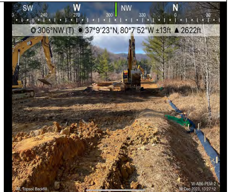
Photo Description: Wetland topsoil restoration
