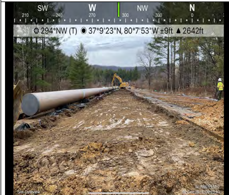
Photo Description: Wetland topsoil removal
