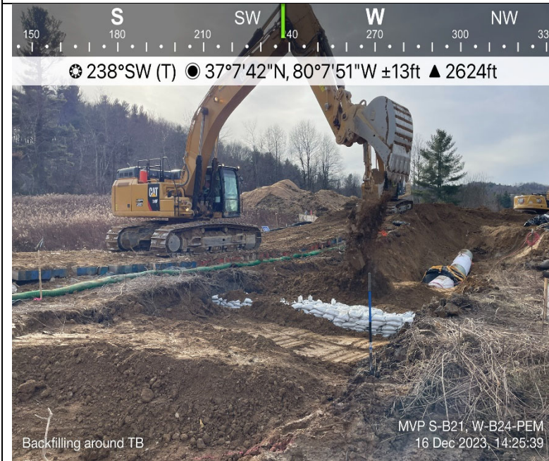
Photo Description: Trenchbreaker installed and subsoil backfill.
