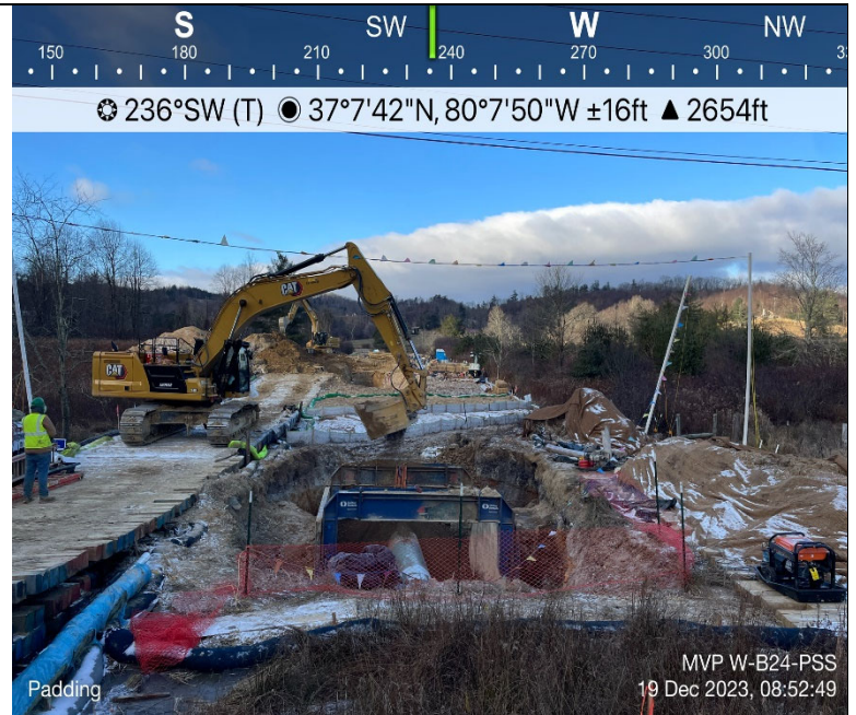
Photo Description: Subsoil padding backfill around pipe.
