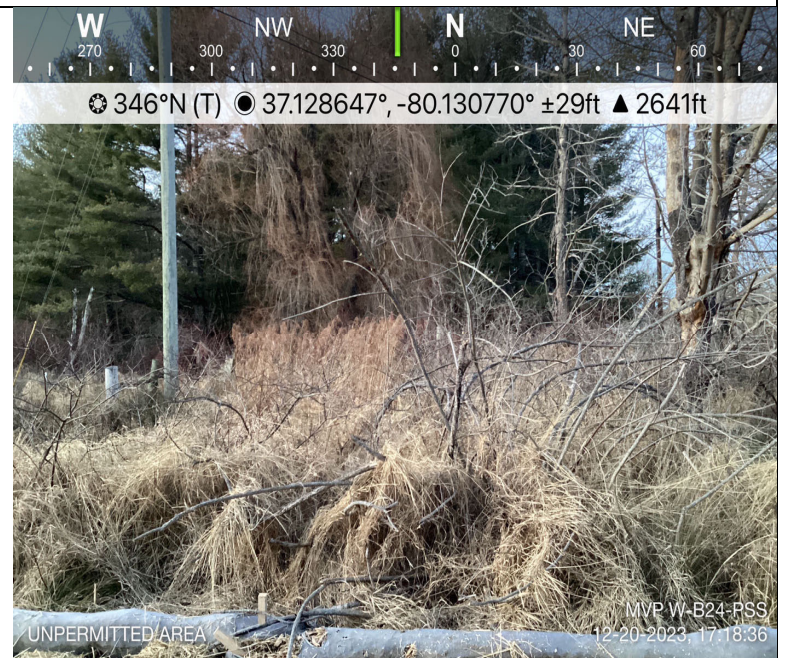
Photo Description: At edge of LOD, view of unpermitted resource area conditions during post-construction assessment.
