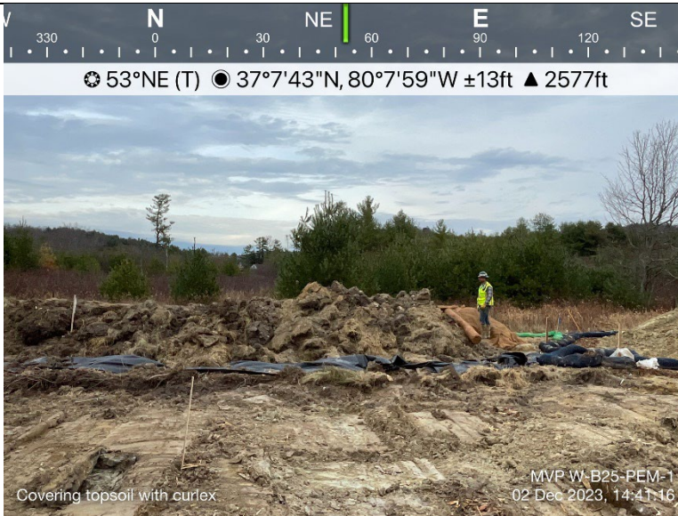
Photo Description: The wetland topsoil in the process of being covered in curlex.
