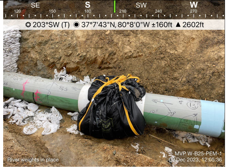
Photo Description: River weights that were installed on the pipe.
