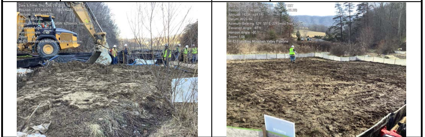
GPS Location See Photo GPS Location See Photo Description Photo 7: Restoring topsoil. Description Photo 8: Seeding aquatic resource.
