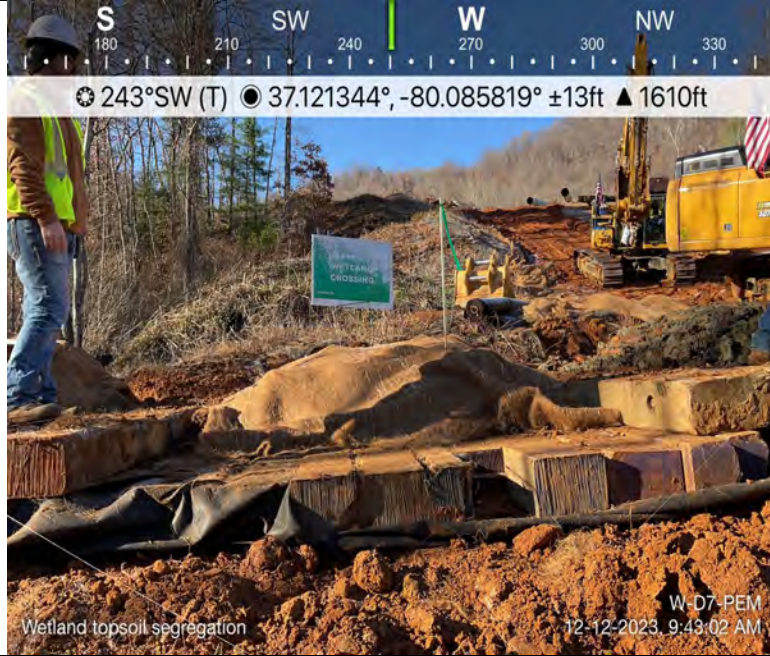
Photo Description: Segregated and stabilized wetland topsoil.
