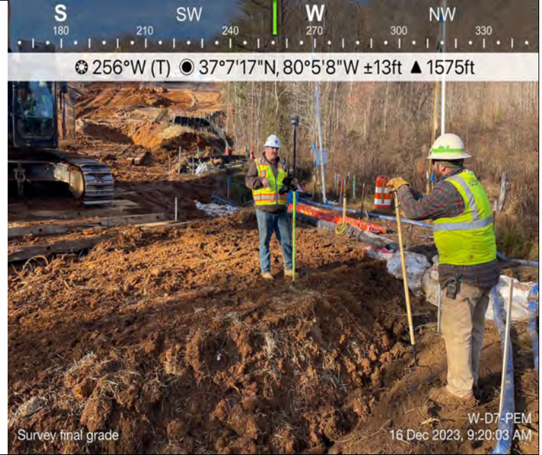
Photo Description: Survey shooting the final grade for wetland topsoil restoration.
