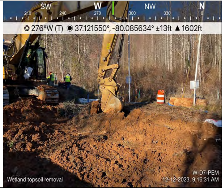
Photo Description: Removal of top 12-inches of wetland topsoil.
