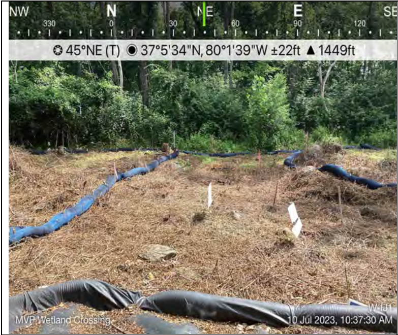
Photo Description: Upstream view of permitted area
