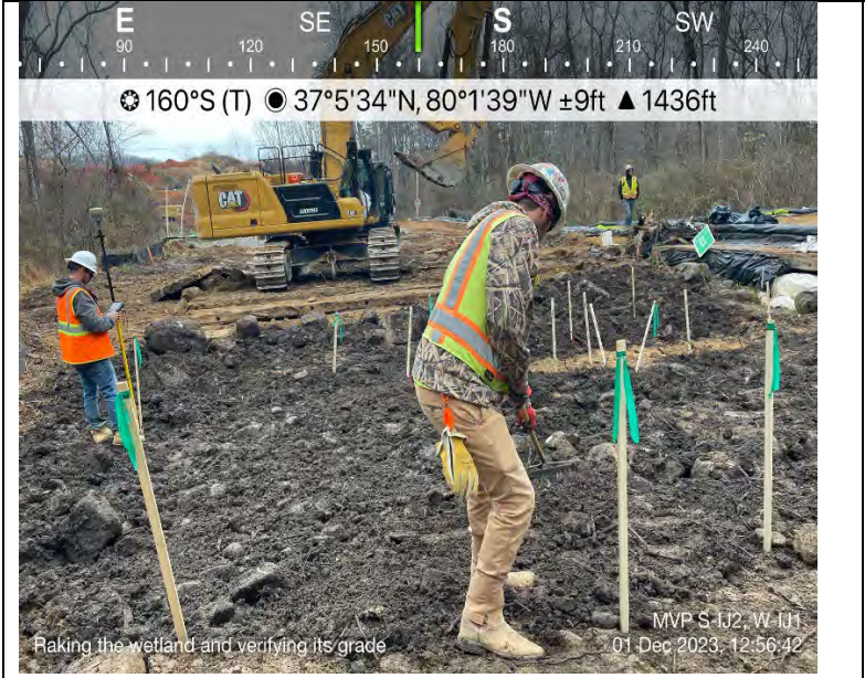
Photo Description: Raking and staking wetland elevations and topsoil.
