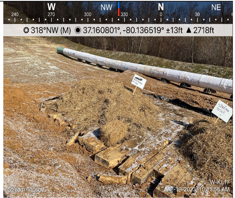
Photo Description: The segregated wetland and stream stockpiles.
