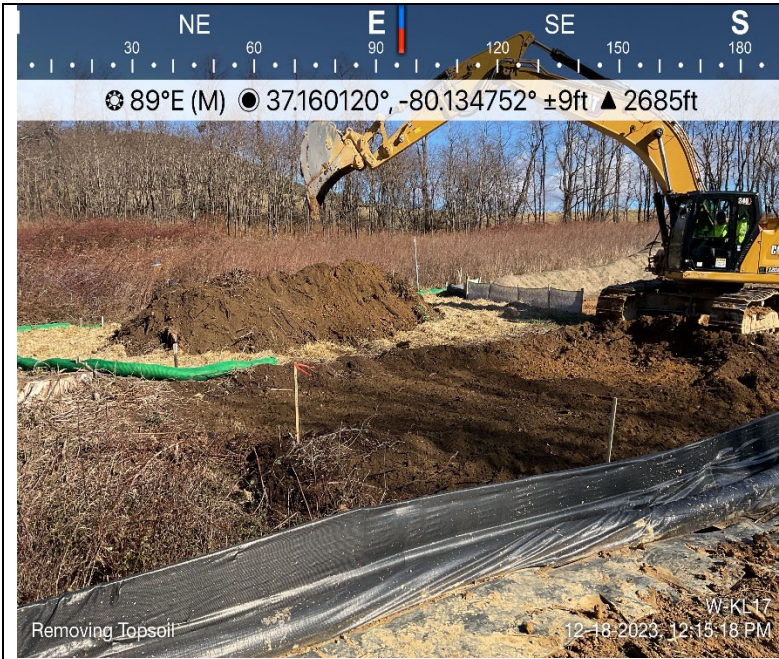
Photo Description: The topsoil was excavated and segregated.
