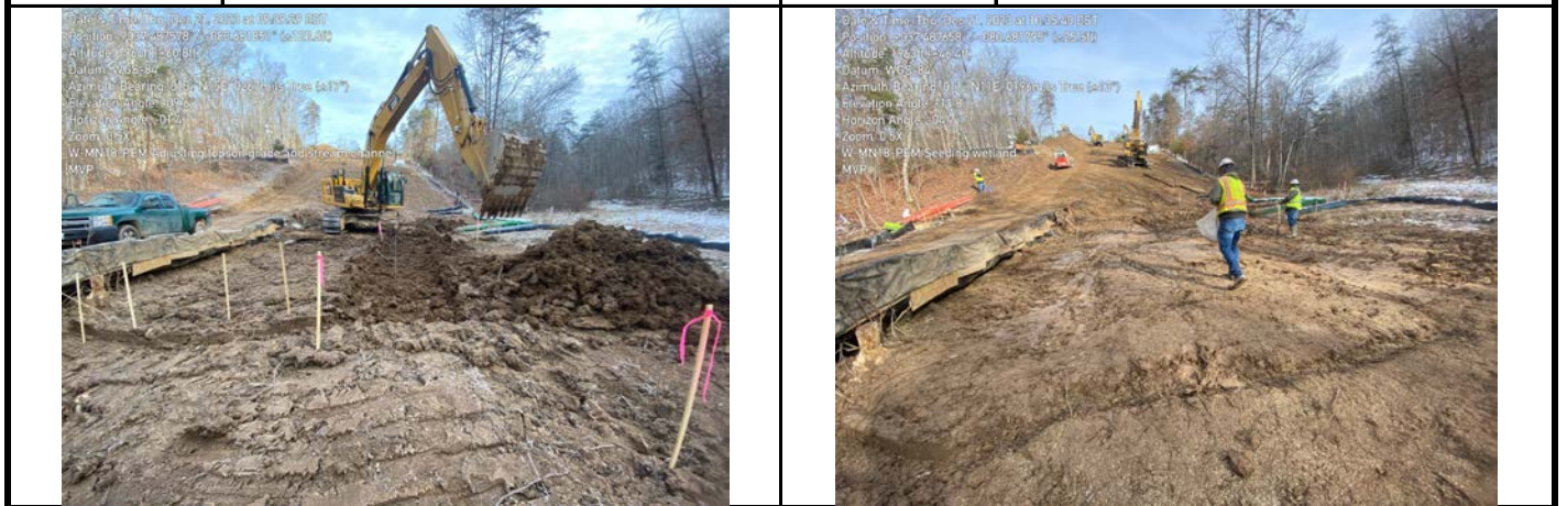
GPS Location See Photo GPS Location See Photo Description Photo 7: Adjusted grade of wetland. Description Photo 8: Seeding wetland.
