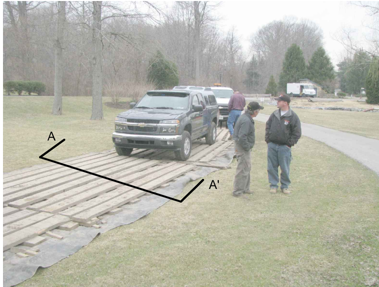
EXAMPLE INSTALLATION USING 10' WIDE DECK MAT
